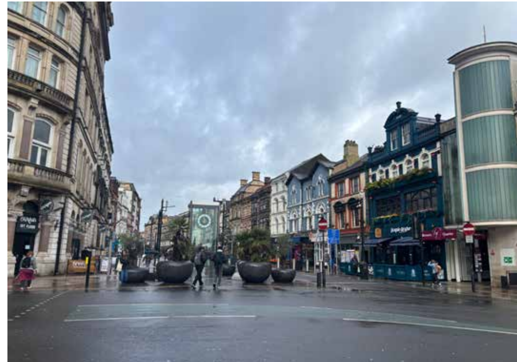
Figure 3.16 St Mary's Street forms the principal route through the centre of the conservation area. It is characterised by its pedestrianised thoroughfare and active streetscape, populated by shopfronts and buildings of varied architectural design, many of which are designated.
