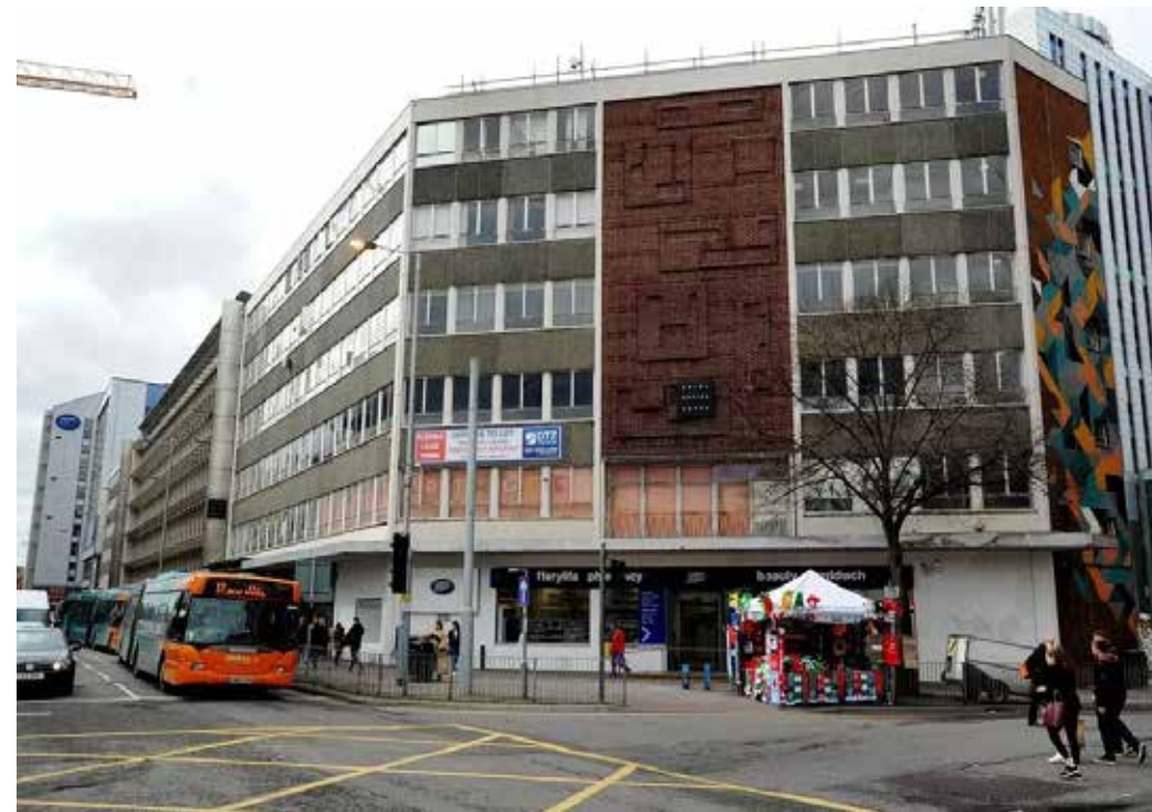
Figure 3.12 2018 Photograph of St David's House Source: Wales Online
