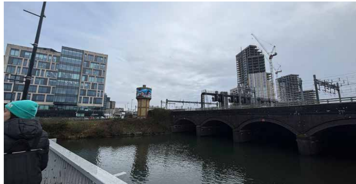
Figure 3.24 View of the Water Tower at Cardiff Central Station (Grade II) from Wood Street Bridge. The Water Tower is experienced in an existing and emerging context of contemporary, large-scale developments.
