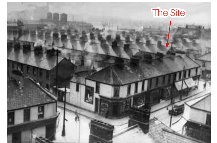
Figure 3.5 1932 Photograph of Wood Street Source: Wales Online
