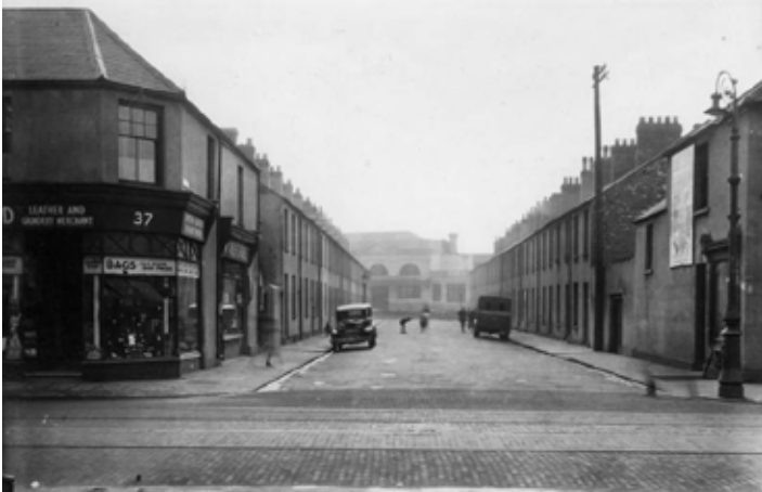
View looking from the application site down Gough Street to Cardiff Train Station
