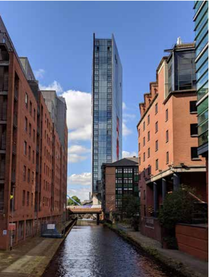
5plus architects, Axis, Manchester
