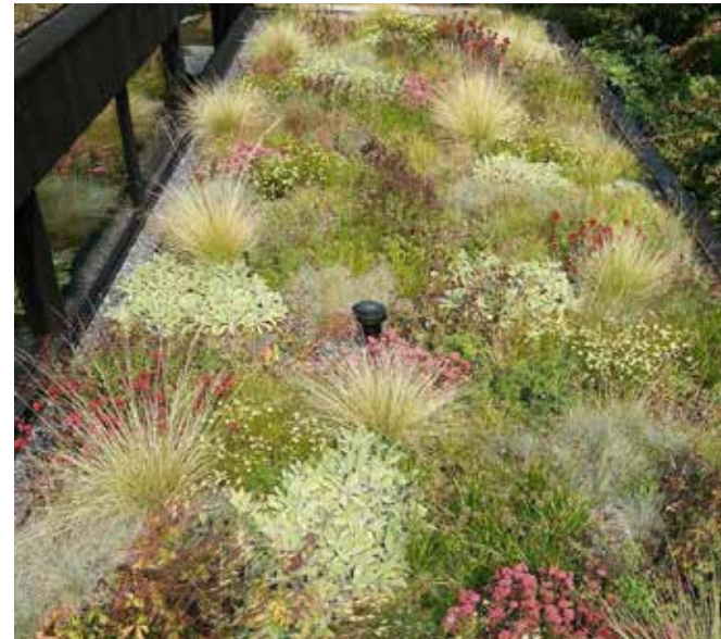
Biodiverse green roofs to support and enhance biodiversity
