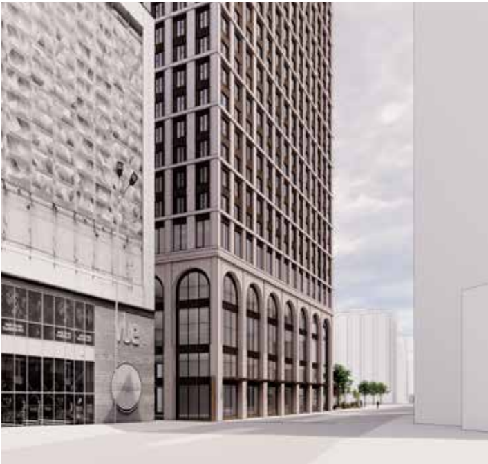
View east down Wood Street
