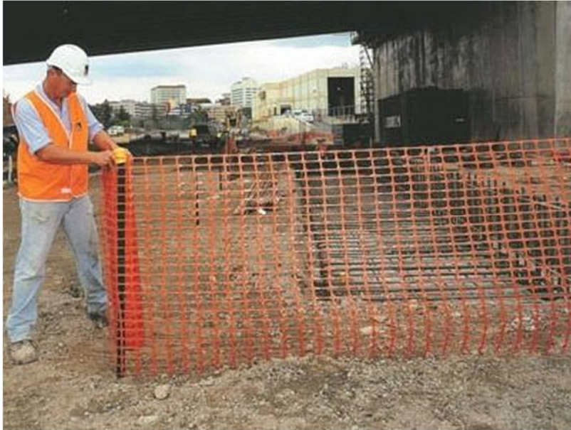
Figure D-4 - Alternative TPF - Example C, plastic mesh with posts
